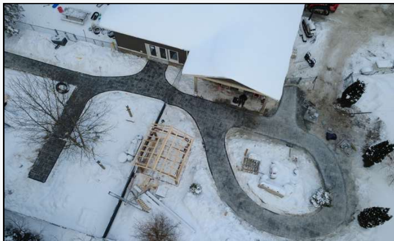
Highlands childcare walkway upgrade
