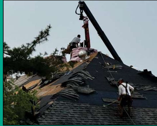
Shingle upgrade (COCHI)
