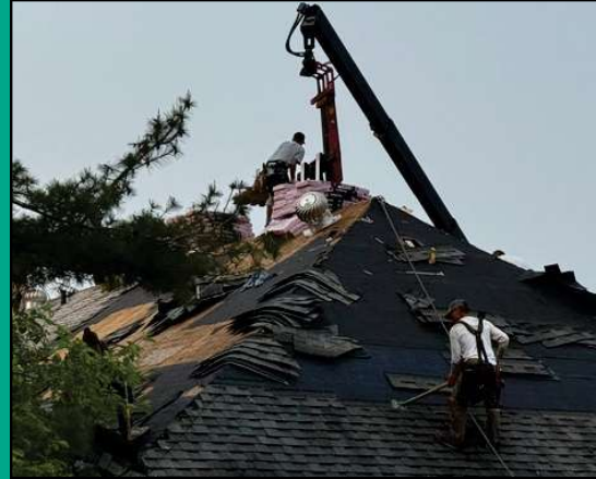
Shingle upgrade (COCHI)
