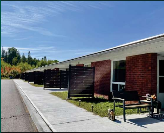
Walkway upgrade (COCHI)
